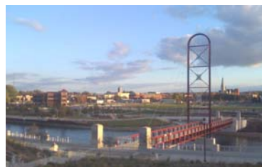
(Riverwalk cable-stayed bridge)
